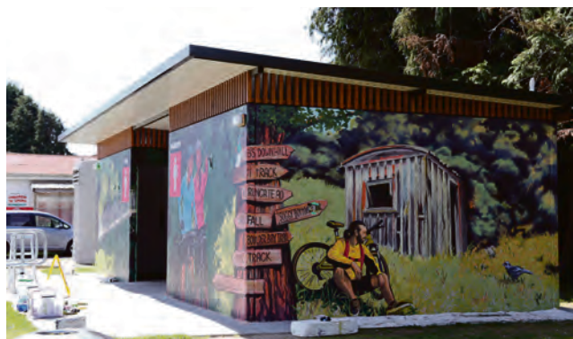
BENNEYDALE PUBLIC TOILETS
