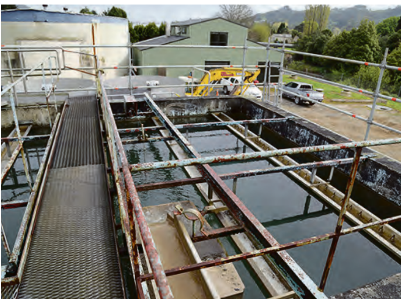
DURING DEMOLITION OF THE OLD BUILDING IN TE KUITI
