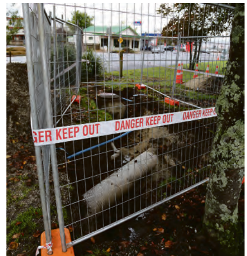
PIPE REPLACEMENT; CARROLL TO RORA ST
