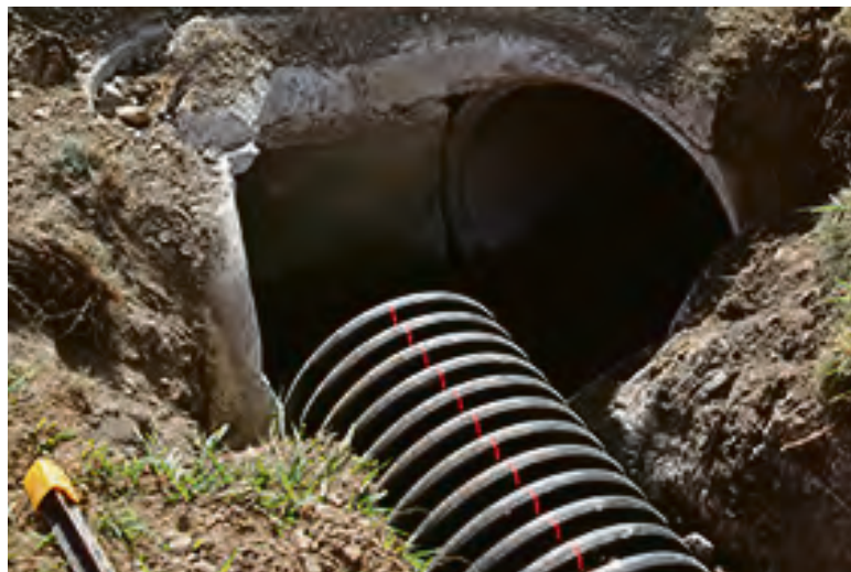
UPGRADE OF STORMWATER DRAIN
