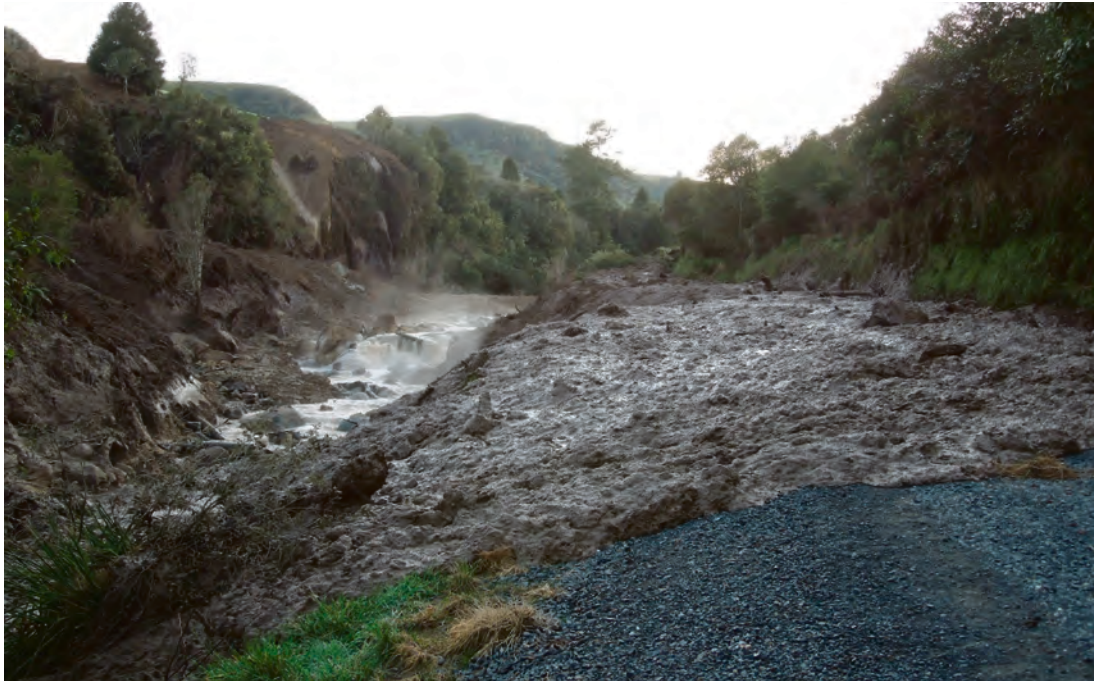
MUD AND DEBRIS AS A RESULT OF SLIP ON MANGAOKEWA ROAD
