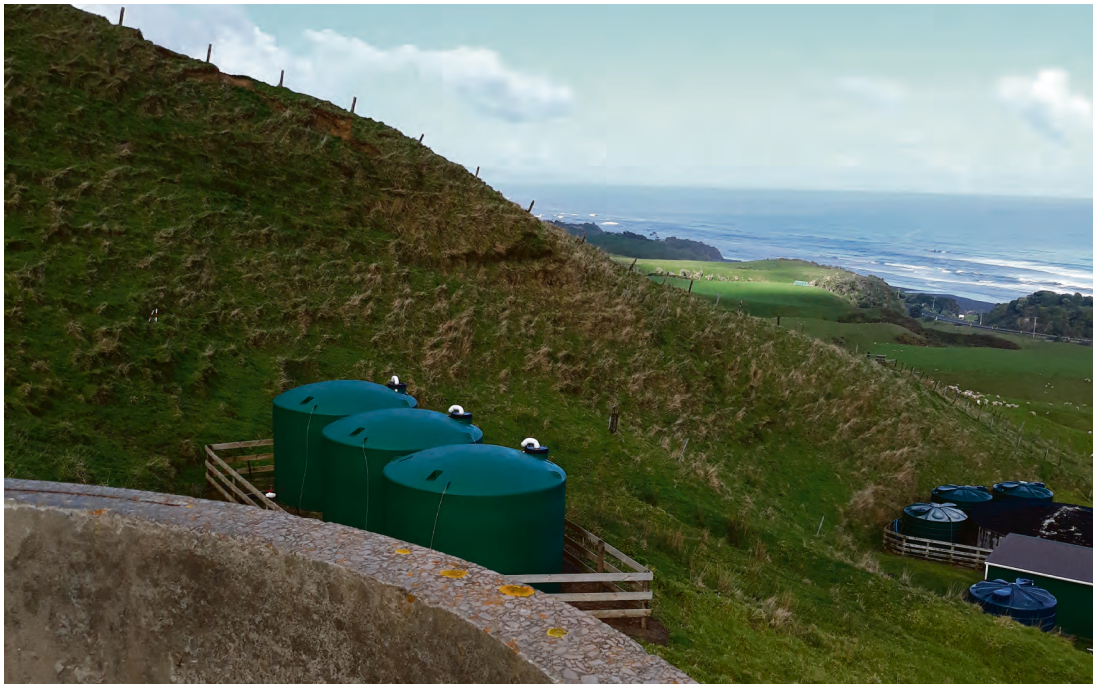
MOKAU WATER SUPPLY - NEW STORAGE TANKS
