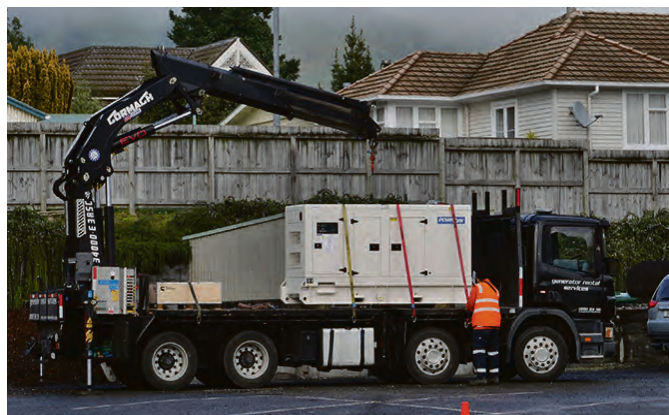
NEW GENERATOR ARRIVES AT WDC
