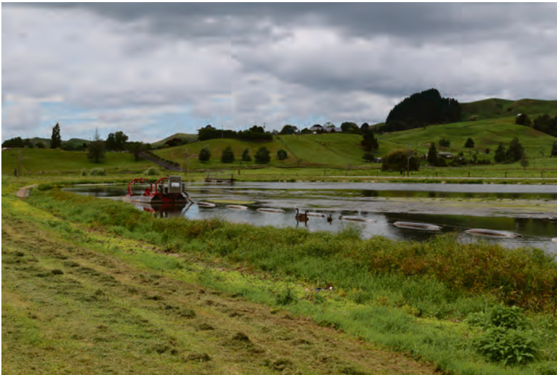
DREDGE LOCATED AT THE TE KUITI WASTEWATER TREATMENT PLANT
